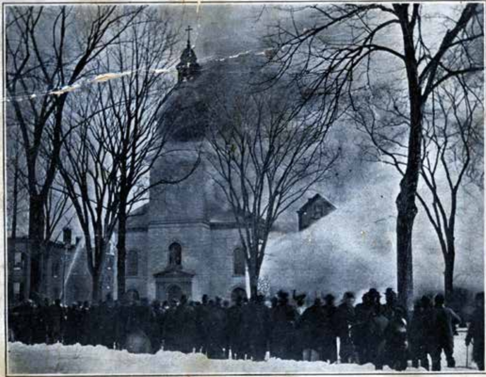
ST. MICHAEL'S R. C. CHURCH. BURNED JANUARY 4TH, 1904.
