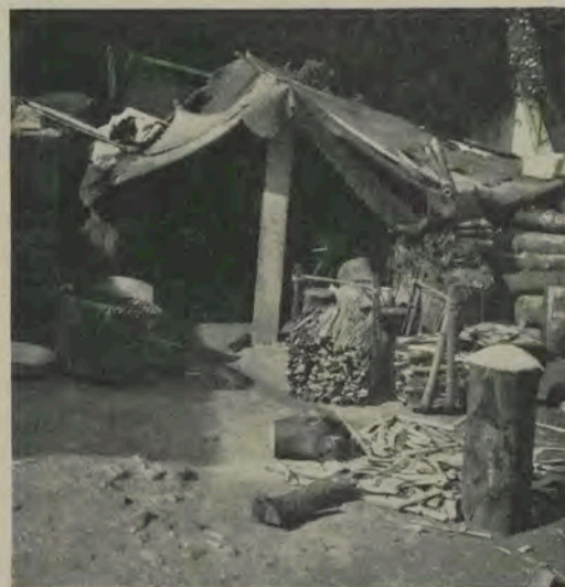
Squatter tent, detail of the above picture
